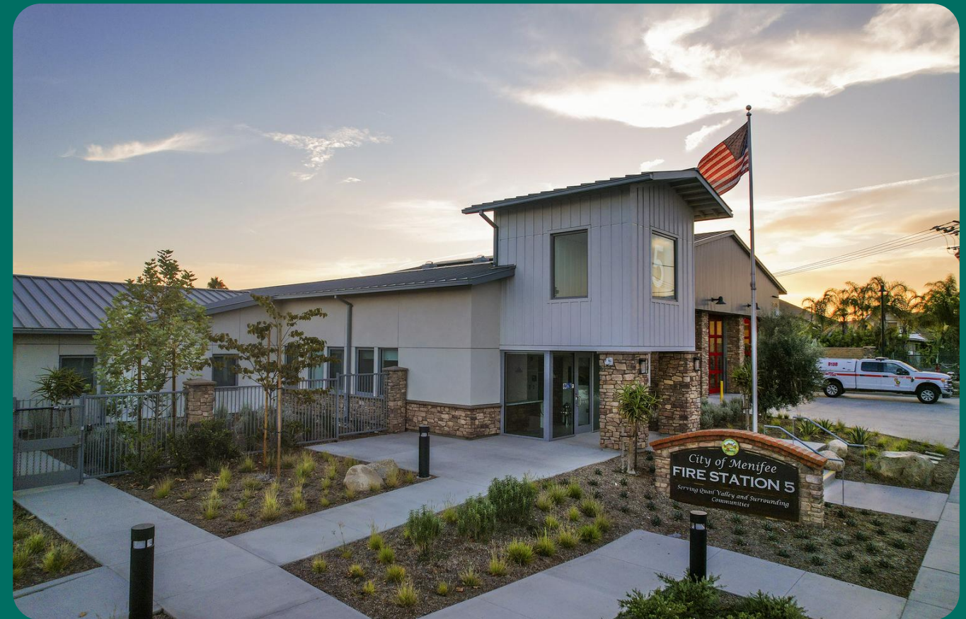
Quail Valley Fire Station utilized light framed wood construction with structural steel to achieve structural performance in a high seismic zone
